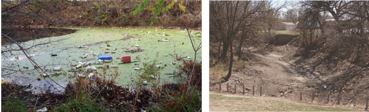
Figure 2: The undersized culverts, accumulated sediments, and lack of flow have led to blighted conditions along the Old Smoky Hill River channel.
